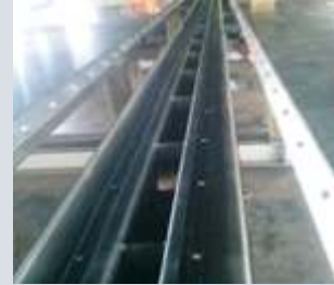
Erection activities of 64 m 2 Horizontal Vacuum Belt Filter at Congo for Copper concentrate application.
