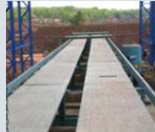
Erection activities of 134 m 2 Horizontal Vacuum Belt Filter at Barbil, India for Iron ore beneficiation application.
