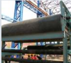
Erection activities of 134 m 2 Horizontal Vacuum Belt Filter at Barbil, India for Iron ore beneficiation application.
